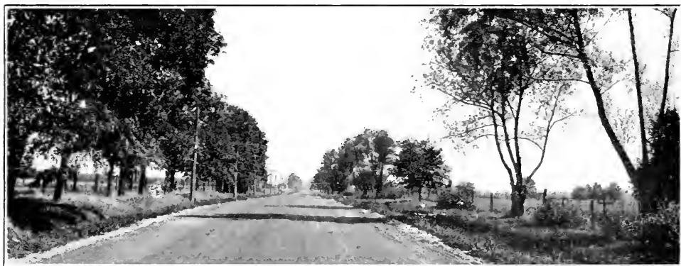
TORONTO-PORT HOPE PROVINCIAL HIGHWAY Gravel surface between Cobourg and Port Hope.
